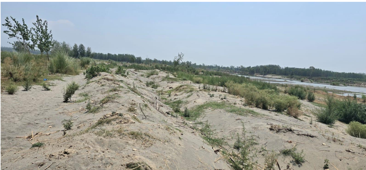
Deposition of Silt at Village Marara Side
