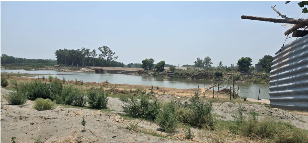
Repair of embankment and removal of temporary roads.
